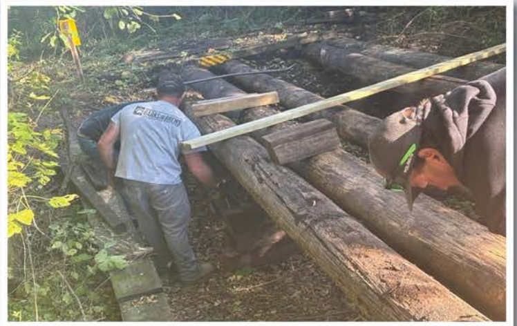
Jacking up telephone poles. Preparing to deck bridge.
