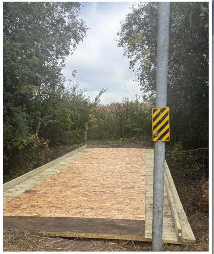
Bridge completed with chip board added to decking
