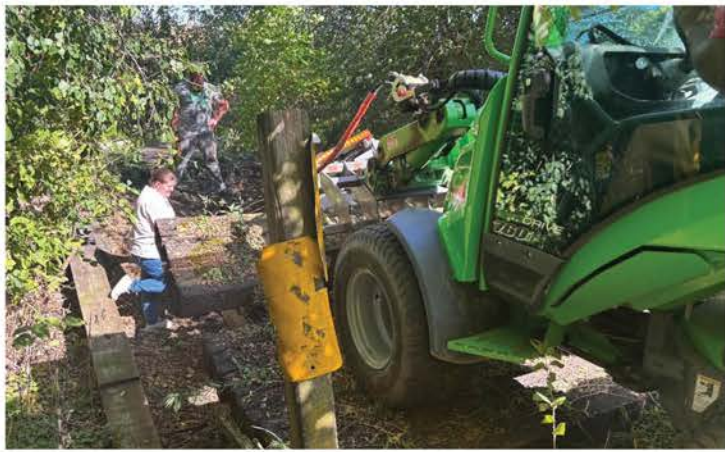
Logging machine removing railroad ties.
