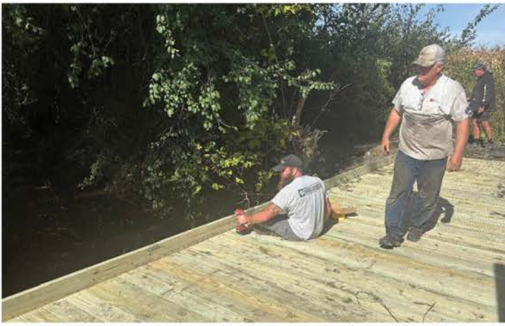
Bridge Decked and Siderails Added
